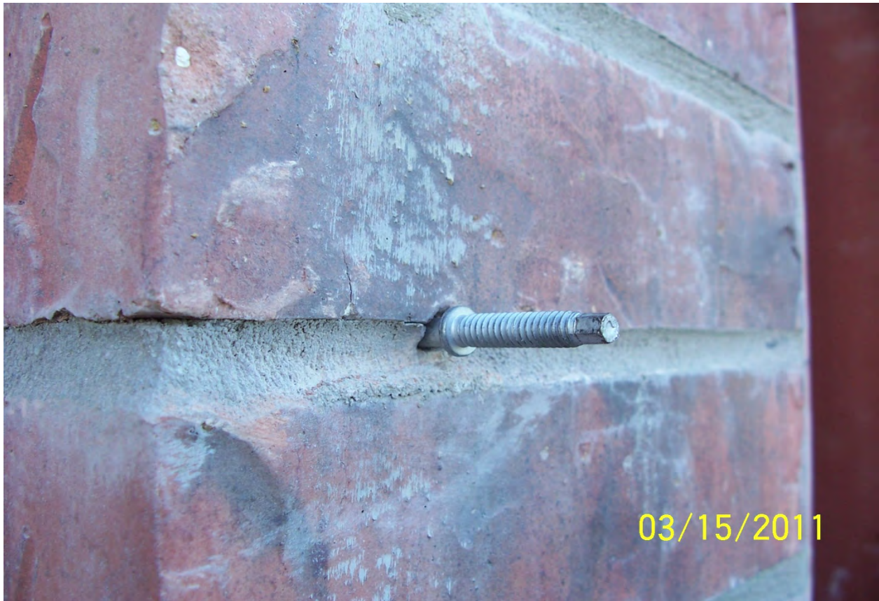
PANELMate PRO TVAS ANCHOR INSTALLED
