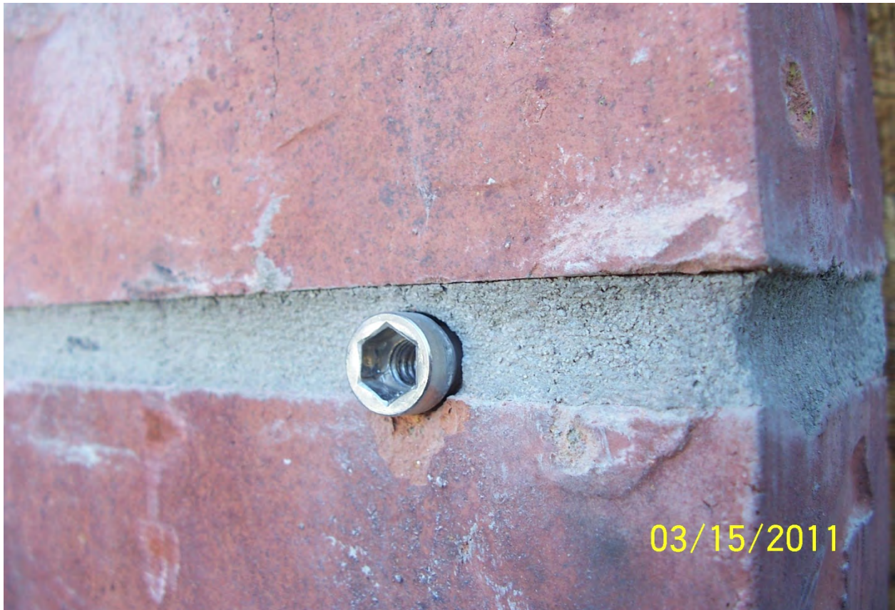
PANELMate FEMALE TVAS ANCHOR INSTALLED
